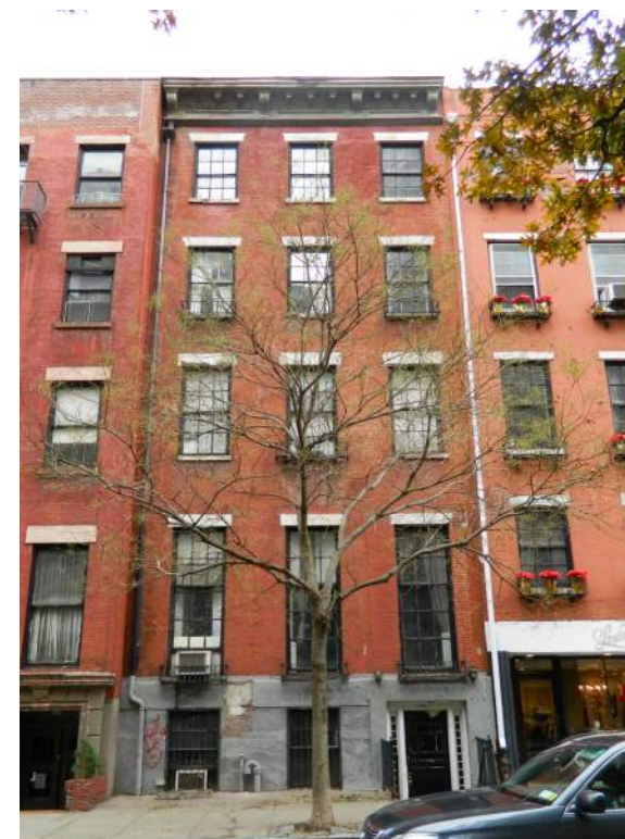
5. LOOKING NORTH FROM E 9TH STREET
