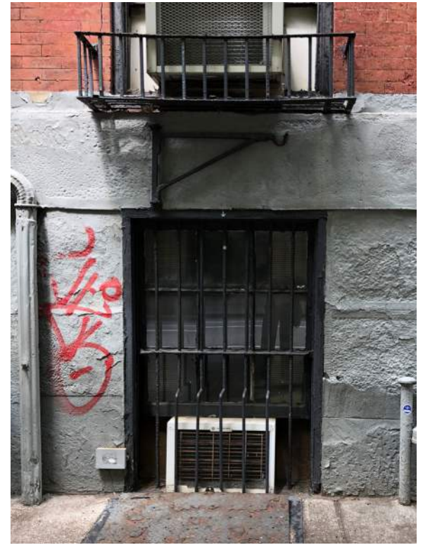
4. EXISTING WINDOWS AT BASEMENT
