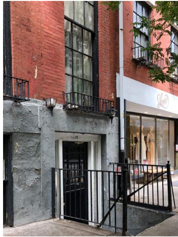
1. EXISTING ENTRY WAY AT E 9TH ST
