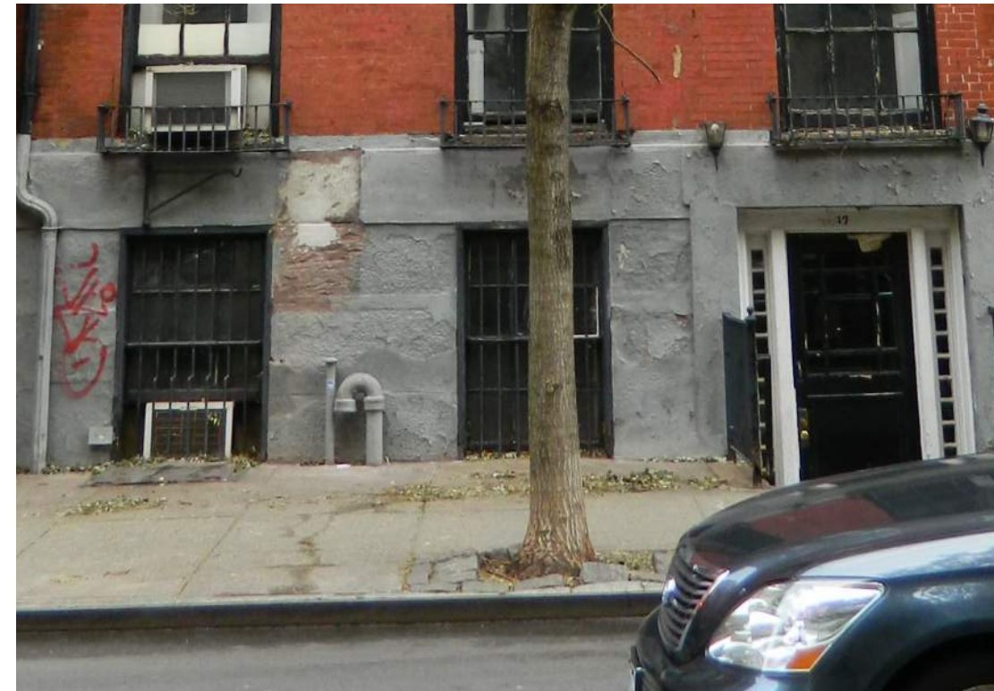
4. EXISTING WINDOWS, BASEMENT
