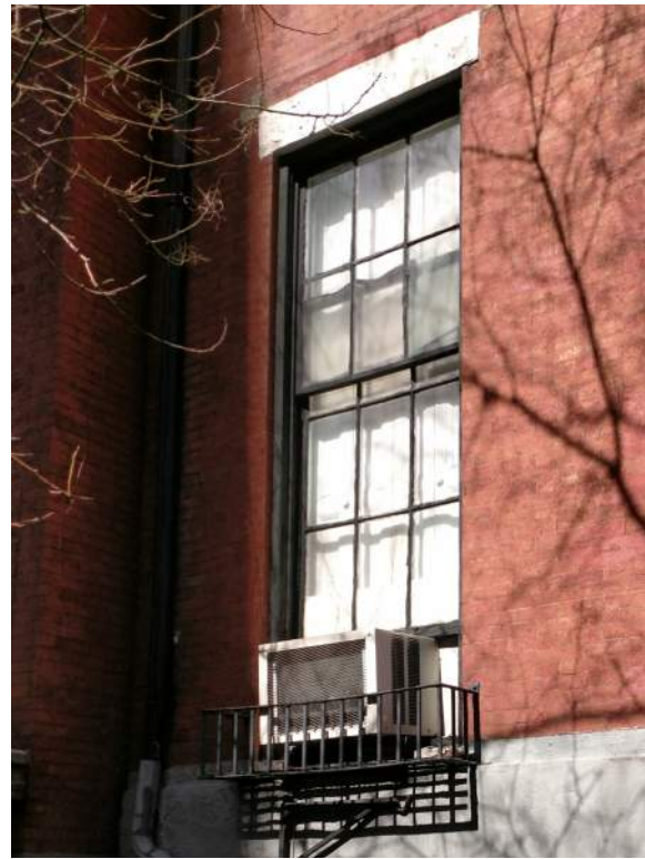
5. EXISTING WINDOWS AT FIRST FLOOR
