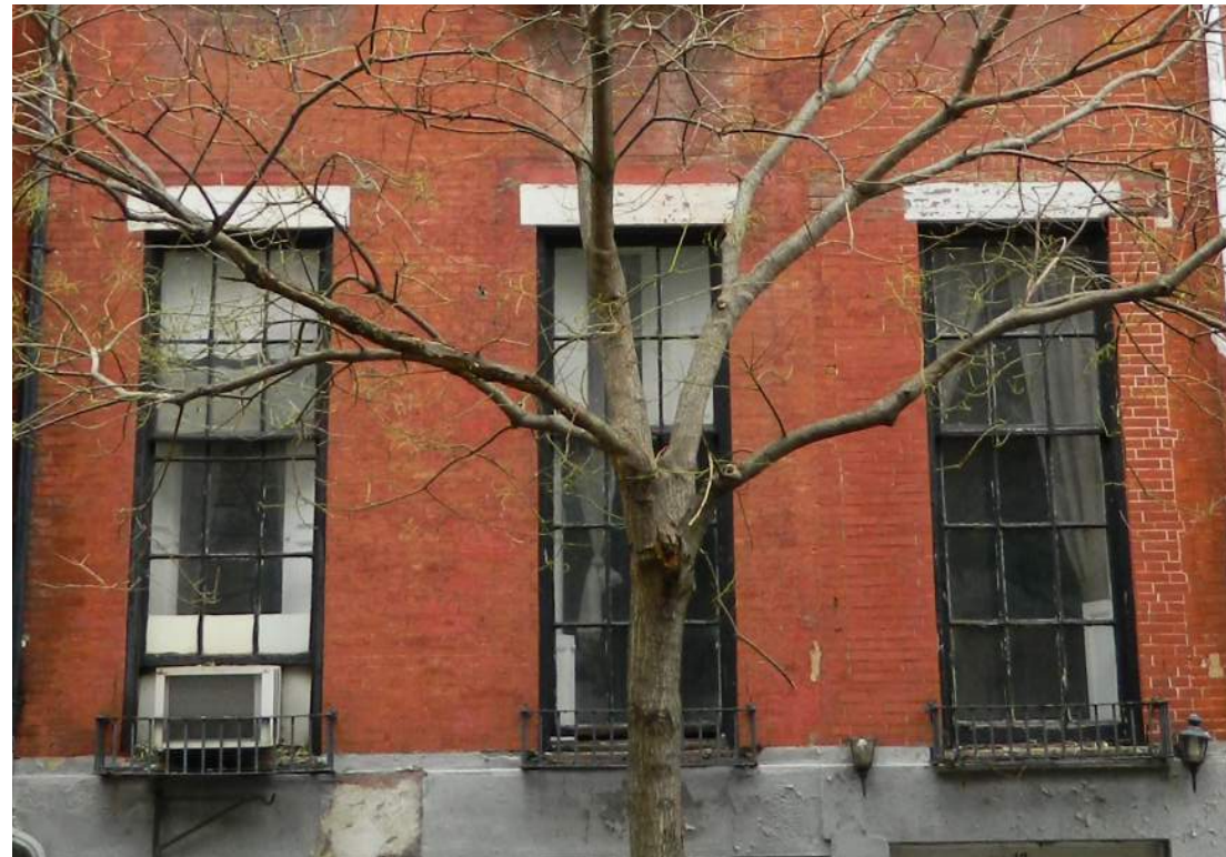
3. EXISTING WINDOWS, 1ST FLOOR
