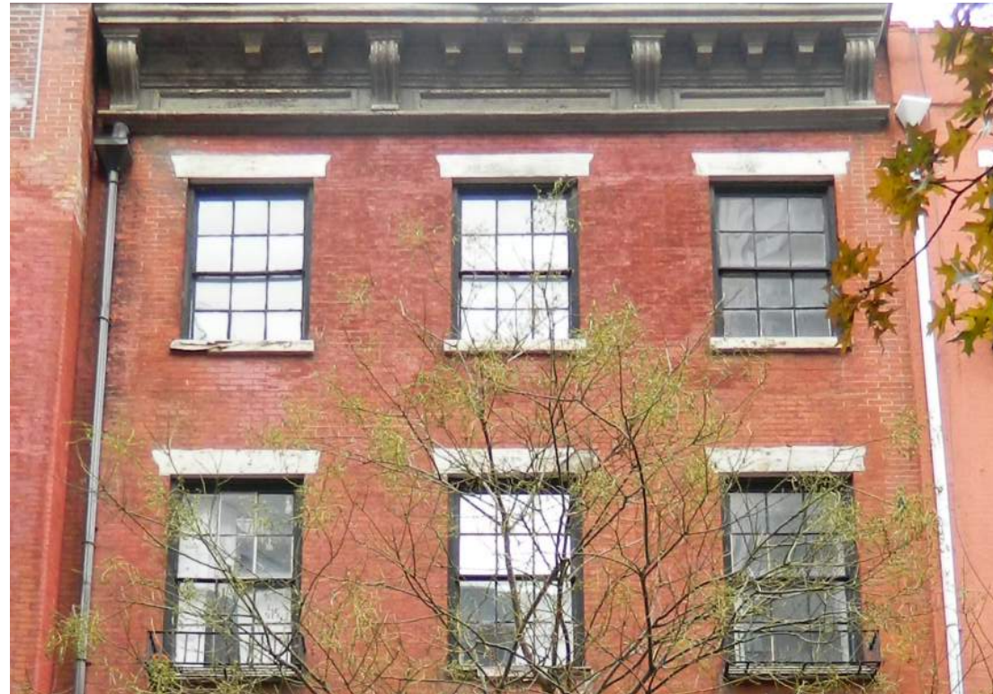
1. EXISTING WINDOWS, 3RD & 4TH FLOORS
