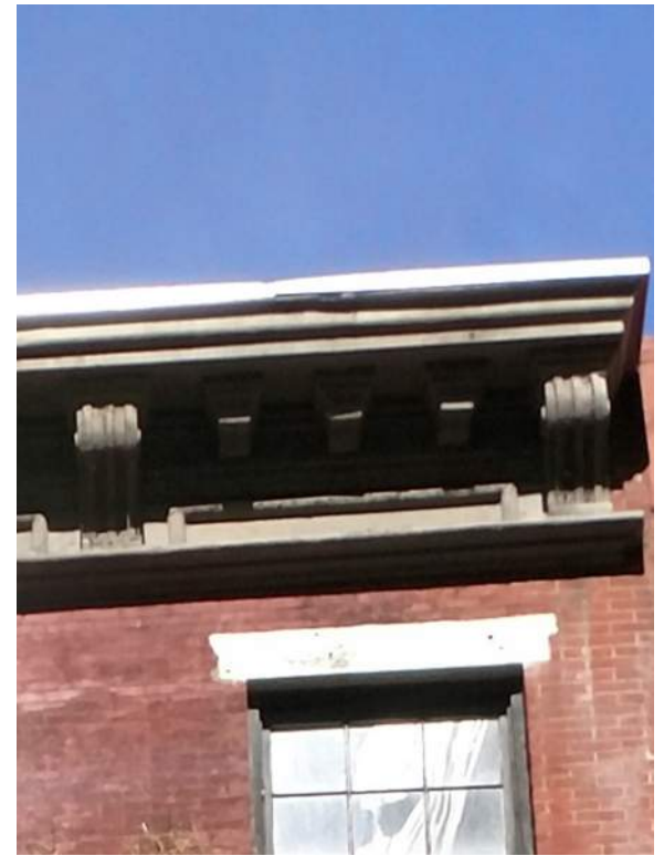
8. EXISTING CORNICE S/E CORNER
