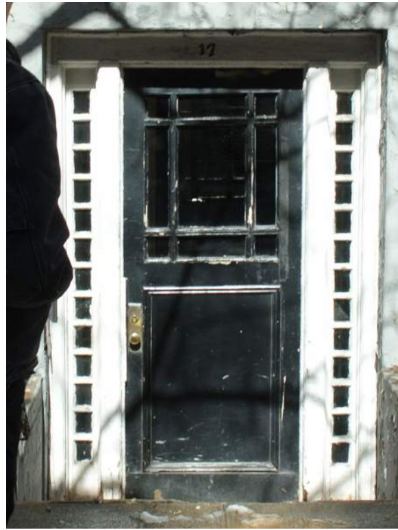
2. EXISTING ENTRY DOOR AT E 9TH ST
