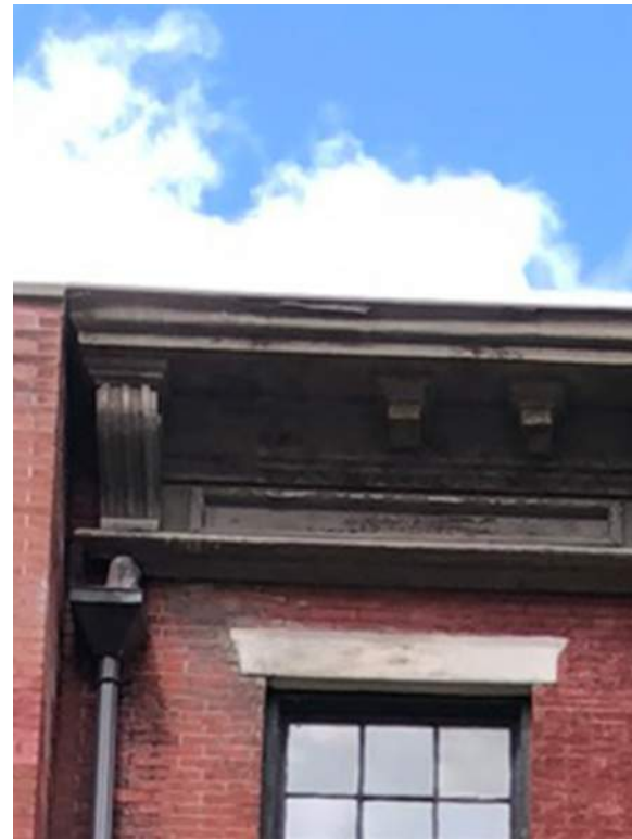
7. EXISTING CORNICE S/W CORNER
