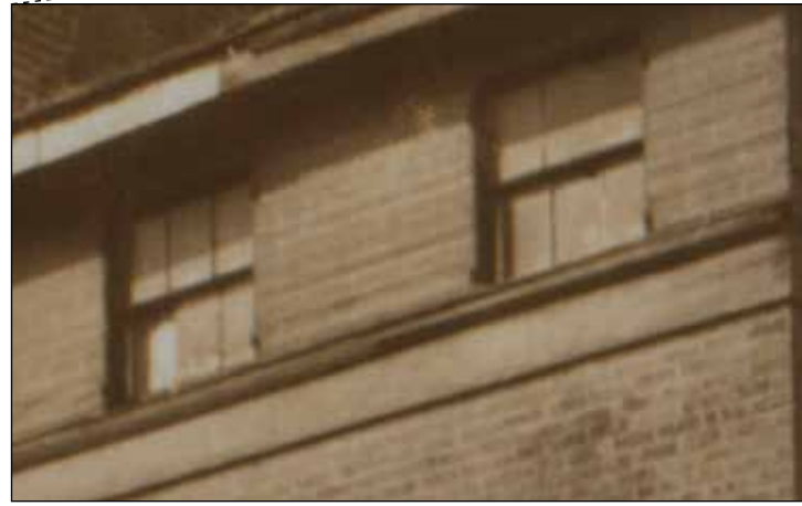
Rooftop Addition Prior to Wood Siding
