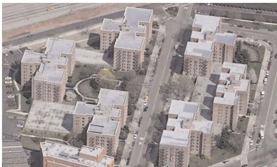
3. Aerial view of the mid-rise residential buildings located east of Linden Place and north of 31st Road.
