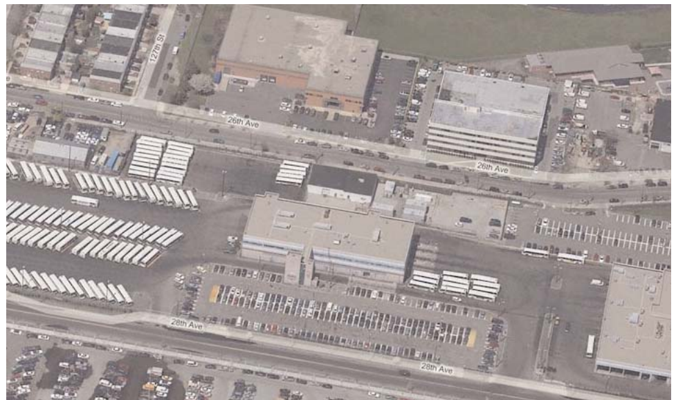
2. A bird's eye view of the MTA bus facility, located immediately to the north of the proposed Academy site.
