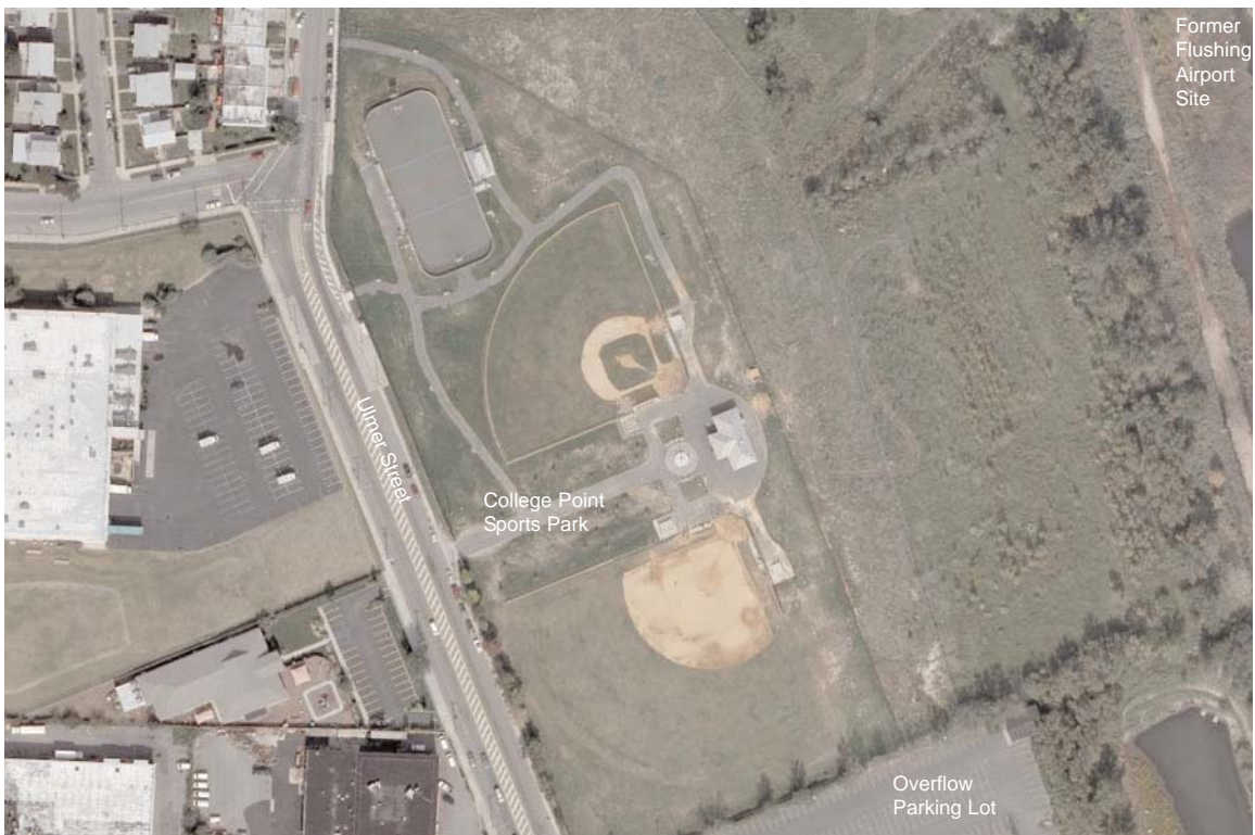
3. An aerial view of the College Point Sports Park.
