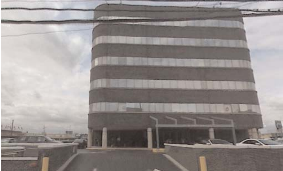
1. Looking west from Linden Place, near 31st Road. This office building is surrounded by an accessory parking lot.
