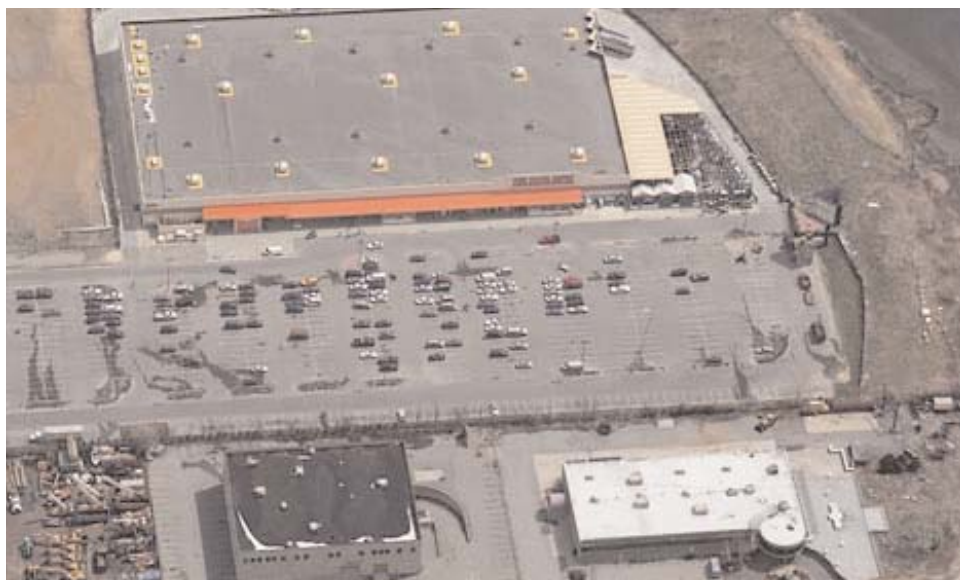
3. A bird's eye view of the Home Depot and accessory parking lot from the west. This is the southern portion of Sub-Area V.
