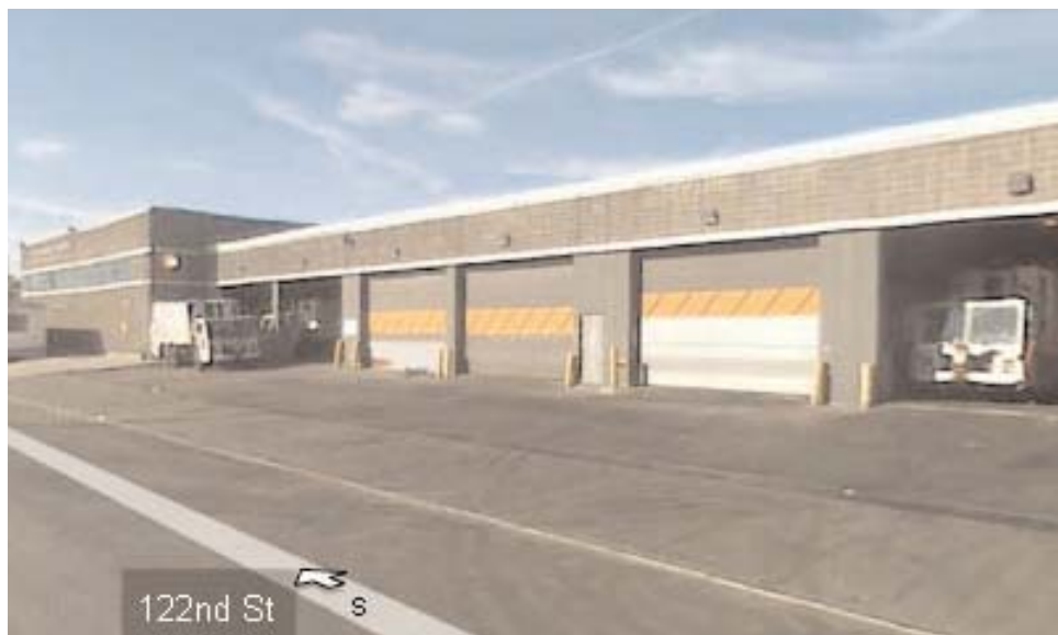
2. A street-level view of the DOS facility. The photograph is taken from 122nd Street looking southwest.
