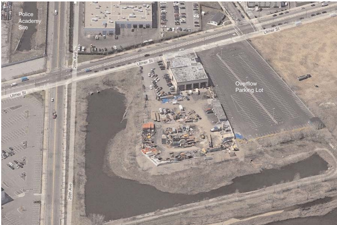
1. A birdseye view from the east of the off-site waterway that is located to the northeast of the proposed Academy site. The waterway is connected to the on-site drainage ditch via culverts that flow diagonally beneath Ulmer Street and 28th Avenue to the proposed Academy site.
