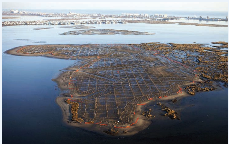
Wetlands Restoration Project, Jamaica Bay
